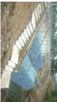
2. Mexborough Road, Adwick on Dearne - Trash Screen Checked before any predicted heavy rainfall events to assess requirement for cleansing.
